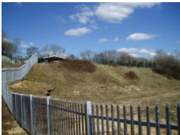
Fig. 6. New protective fence at Horn Park Quarry, Dorset, SW England.
